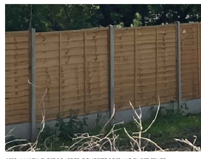
1800MM HIGH CLOSE BOARDED CONCRETE POST AND TIMBER FENCE
